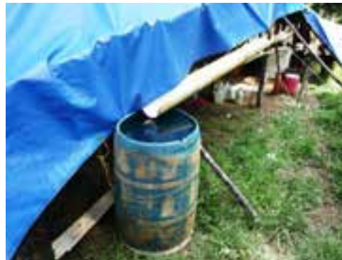
Local rainwater collection system
